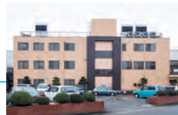
Sakana Machi Hospital
